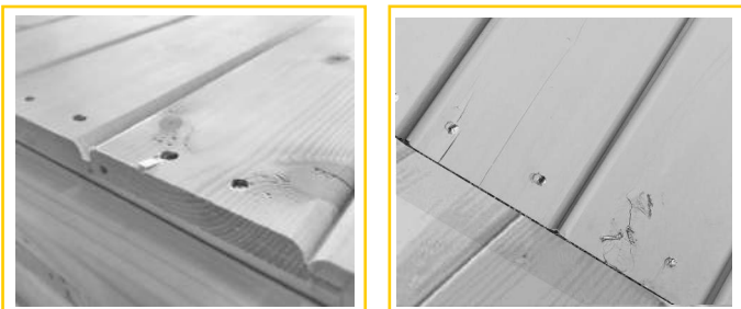
Examples of nailing and nail heads :
