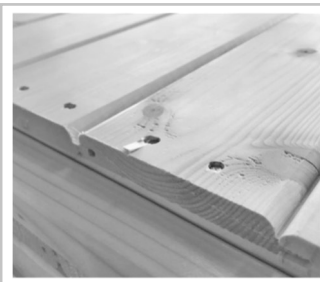
Examples of nailing and nail heads :
